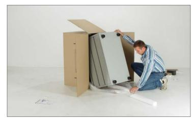
10. Tilt the cabinet back and slide the foam strips under the cabinet as far as possible. Space them between the wheels so they won't be in the way when the cabinet is righted.
